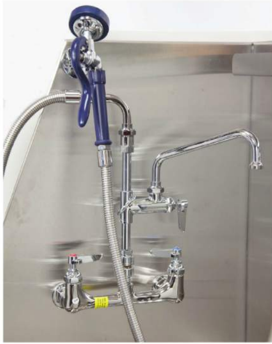
Spray valves used in multi-family settings should be heavy-duty. A utility spigot can be provided if there is not a sink in the pet care room.
